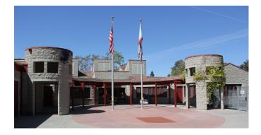
Carmel Del Mar School was constructed in 1991. It is a single story school with one main building with additional relocatable classrooms. The primary material in the permanent buildings is split face concrete block walls with drywall interior finishes. There is a combination of flat and sloped roofs.
