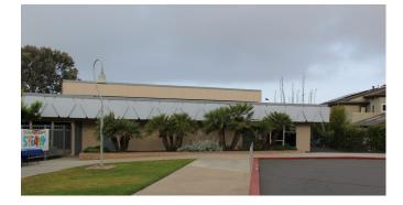
Del Mar Heights School was constructed in 1959 and is the oldest site within the District. It is a single story school with multiple hexagonal buildings and additional relocatable classrooms. The primary material in the permanent buildings is plaster with drywall interior finishes. Roofs are flat, built up with gravel ballast. Hexagonal metal panels surround the buildings' fascia in an attempt to provide shade.
